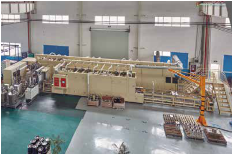
Auto-assembly Line for Vacuum Pouring of Epoxy Resin
